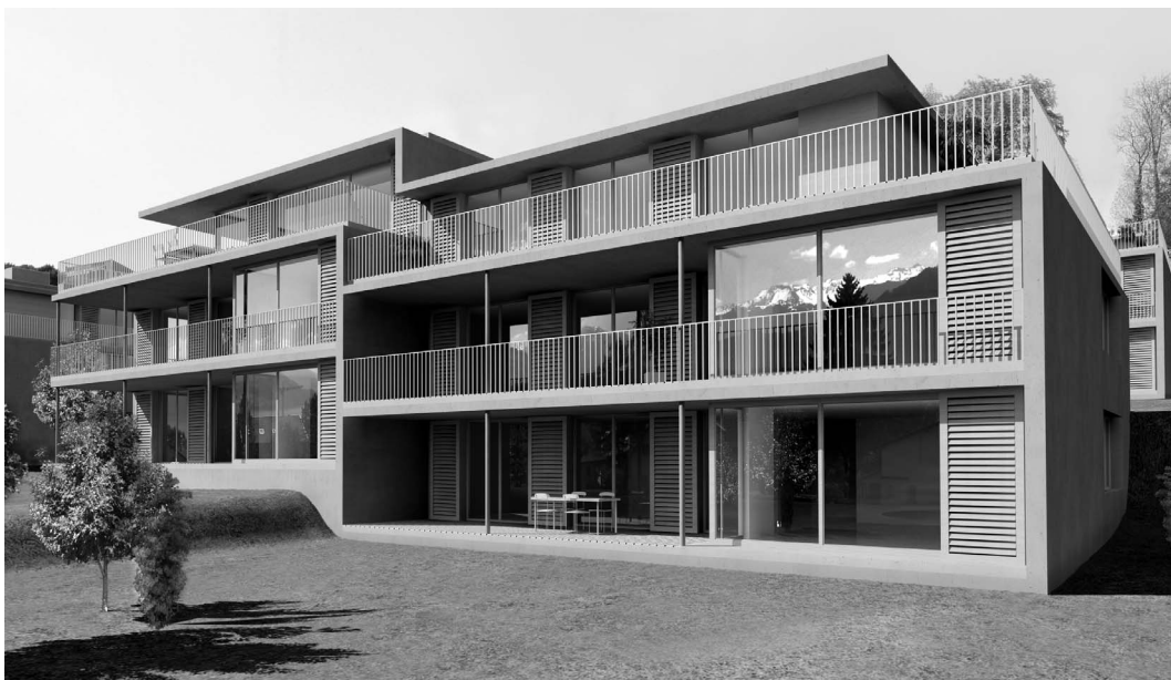
Example stacking 90° to the slide axis: The shutters run in front the parapet and provide shade on the balcony.
